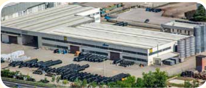
Production Centre - Imola (BO) - Italy
